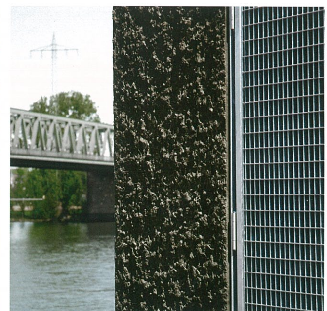
Die Oberfläche ist bis zu 30 Millimeter tief 'gespitzt' behauen. | The surface has been textured with dents up to 30 millimetres deep created by pointed chisels.
